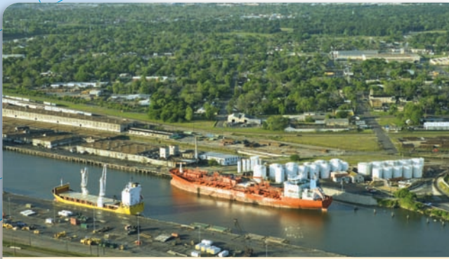
2 Large white containers, shown here at the Port of Houston, store oil from the Gulf Coast.
